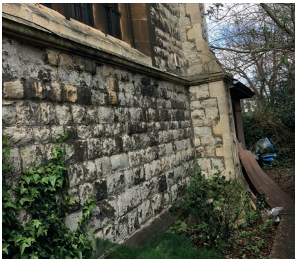
g. South transept elevation - low level.
