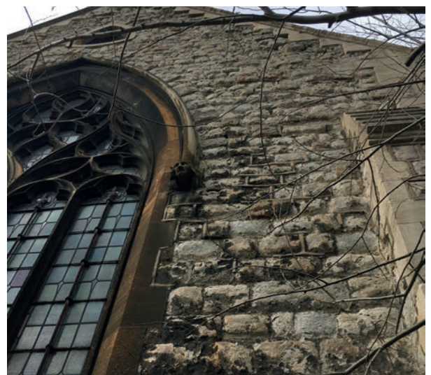
f. Overview of south transept elevation.
