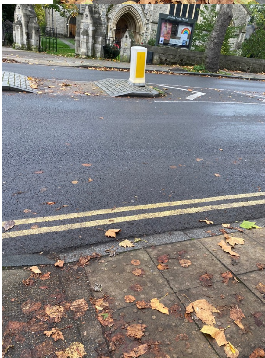
Figure 2: Dropped kerbs provide easier access from the pavement opposite the church
