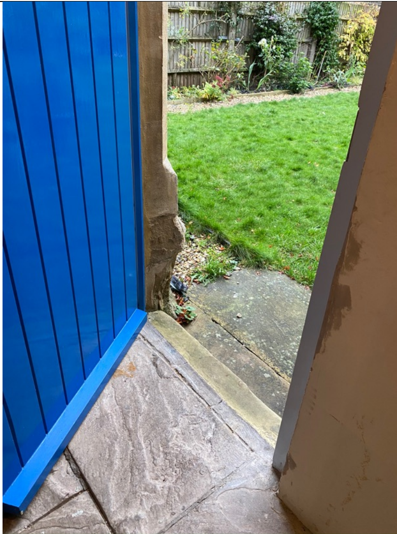
Figure 9: Small step down from the sanctuary to the garden is uneven and hard to see - could cause someone to trip. Avoid using and mark with yellow tape
