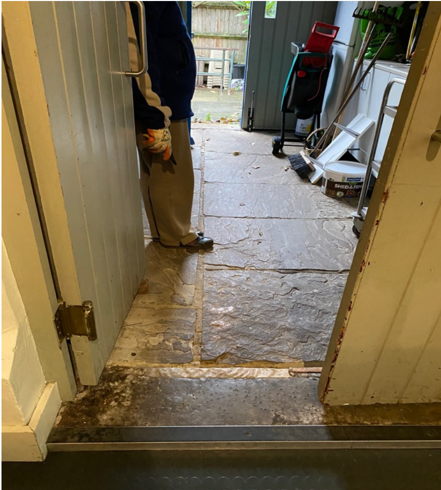
Figure 8: Step from the kitchen out towards the garden is hard to see and needs a yellow strip
